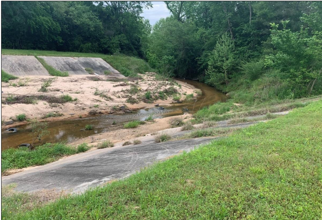
Figure 16. View of Stewarts Creek South of Silverdale Drive Bridge (Facing Southeast)
