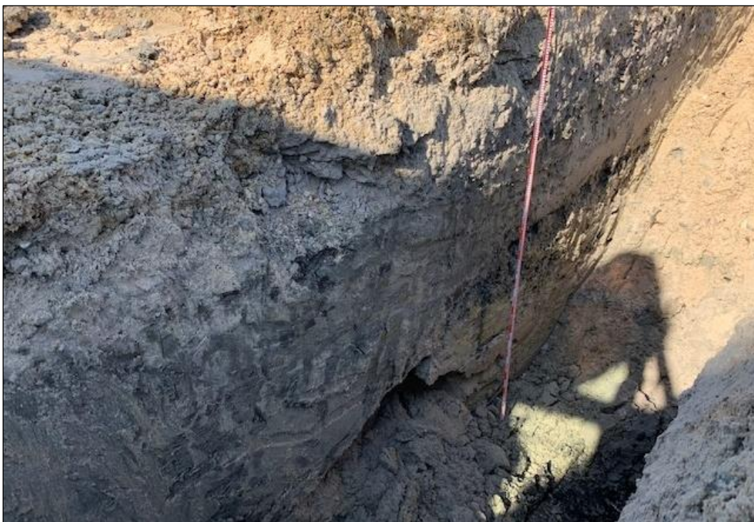
Figure A-12. Overview of THT-4 (Depth of 2.0 Meters)
