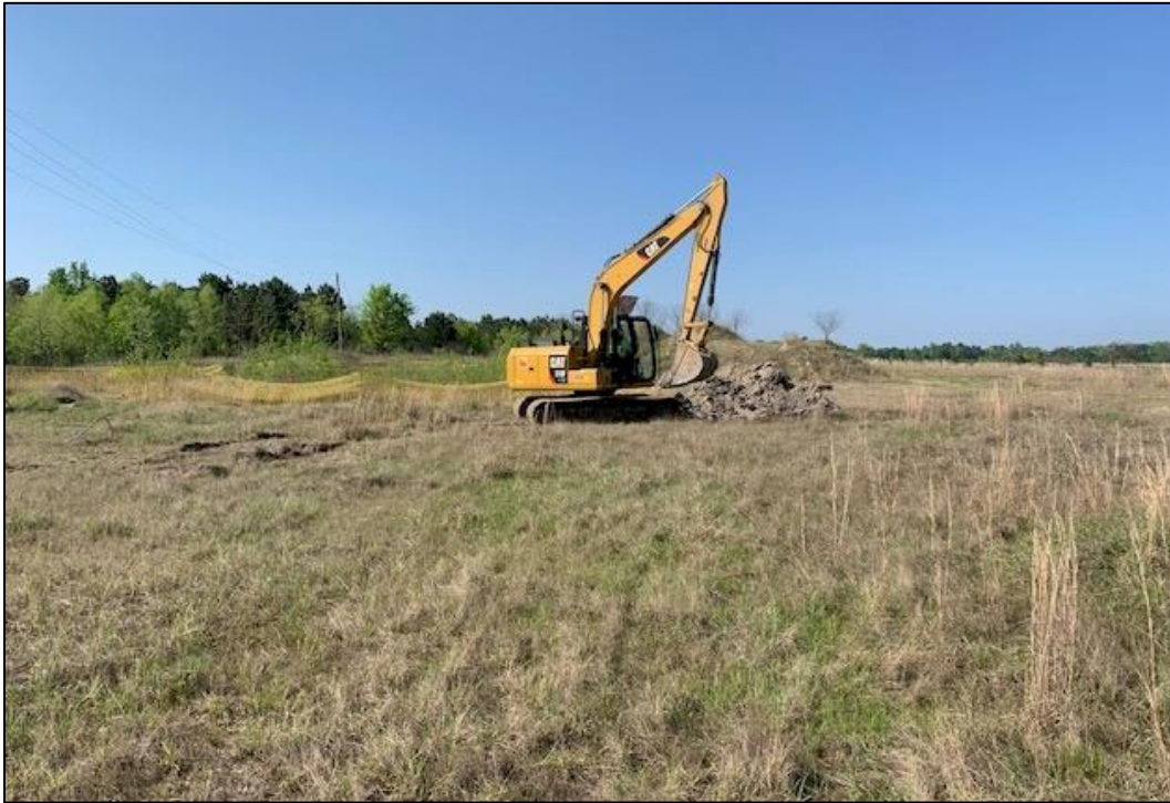
Figure A-11. Overview of Location of THT-4 (Facing North)
