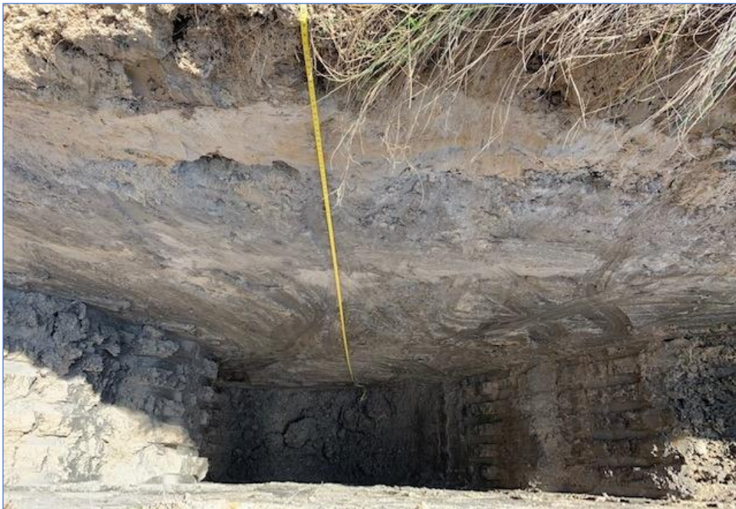
Figure A-4. View of Final Excavation of THT-1 (Depth of 5.5 Meters)
