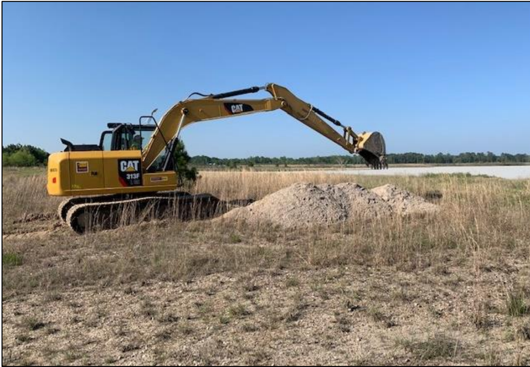
Figure A-14. Overview of Location of THT-5 (Facing North)
