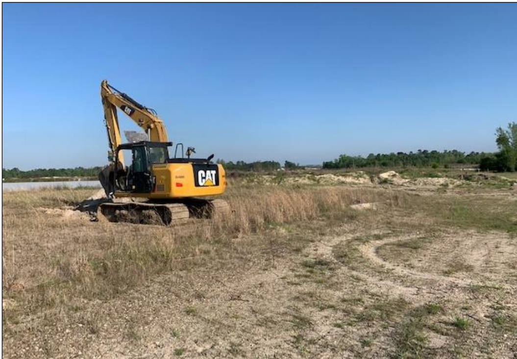
Figure A-17. Overview of THT-6 (Facing Southeast)
