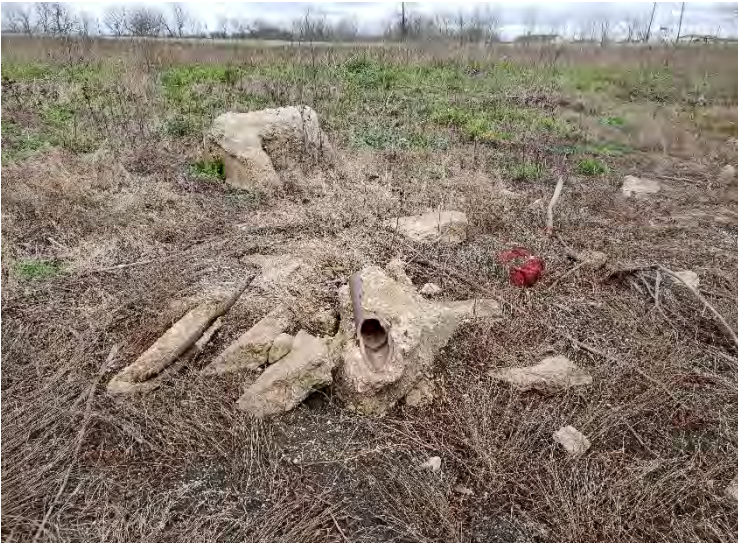
Photograph 13 – Inline PS APE, concrete debris in wetland, view to the northwest.
