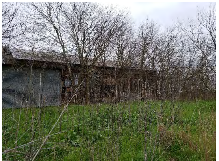
Photograph 12 – In-line PS APE, modern barn, view to the southeast.
