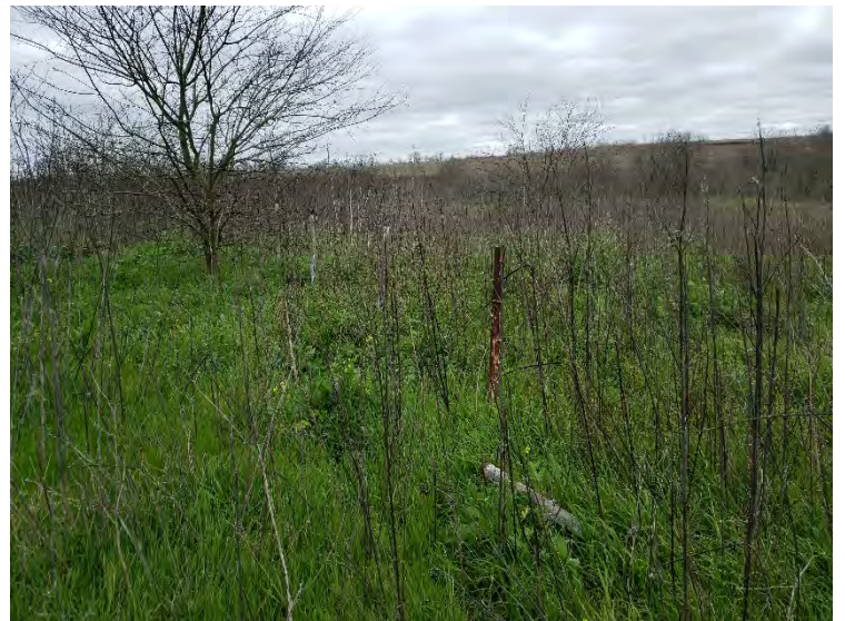
Photograph 6 – In-line PS APE, general setting, metal pipe fencing, view to the southwest.
