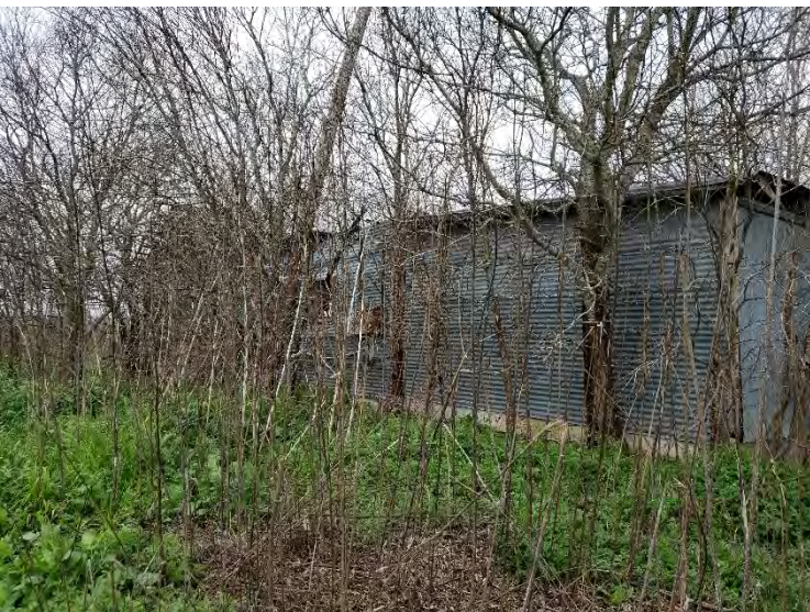
Photograph 11 – In-line PS APE, modern barn, view to the northwest.
