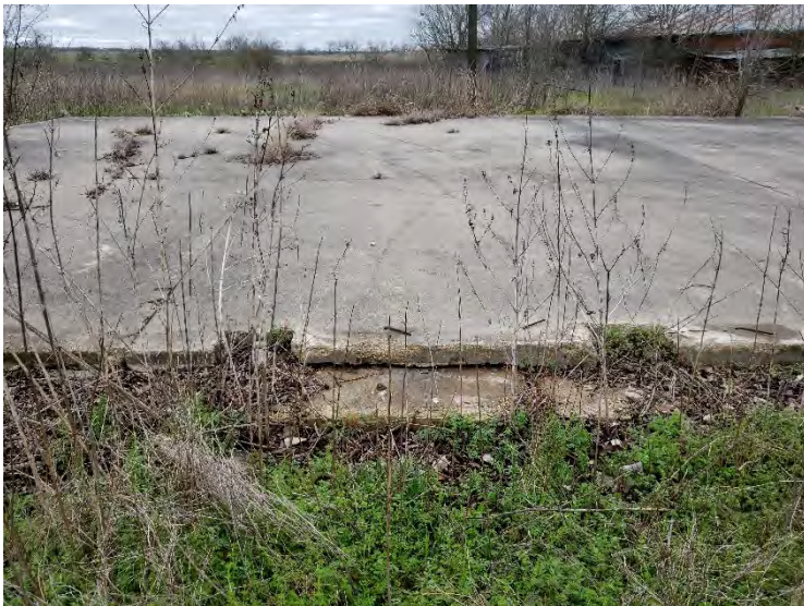
Photograph 35 – 41WM1419, Feature 1, view to the southwest.
