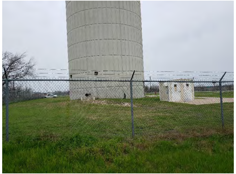
Photograph 20 – Frame Switch PS APE, view to the west.
