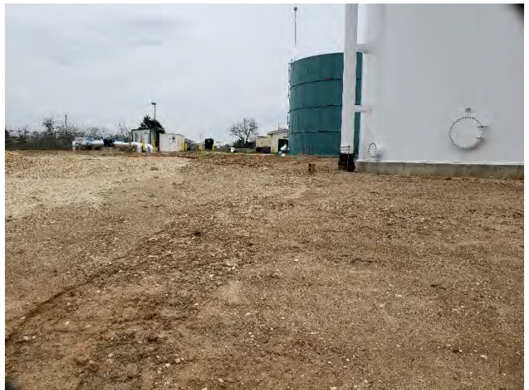
Photograph 24 – Shiloh PS APE, recent ground disturbance, view to the southeast.
