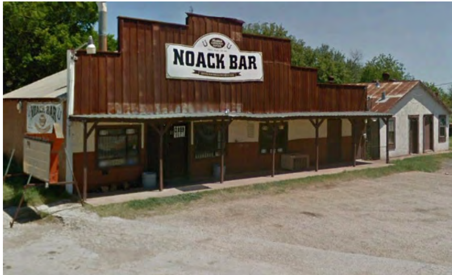
Photograph 3 – AR-3, 7401 FM 112, view to the northeast.
