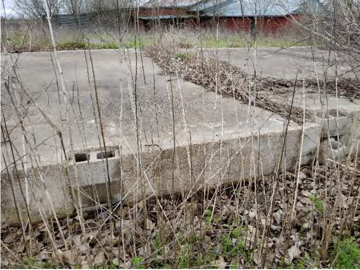
Photograph 38 – 41WM1419, Feature 1, view to the southwest.
