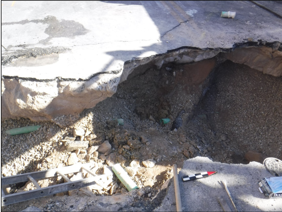
Figure 5-4. Disturbances observed during the excavation of the main trench; facing northwest.
