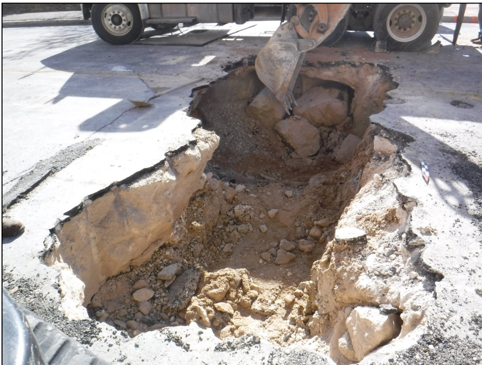
Figure 5-5. Typical profile of the main trench; facing south
