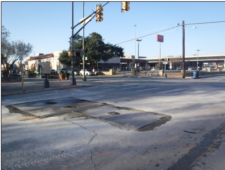
Figure 5-3. Overview of the Area of Potential Effects; facing southwest
