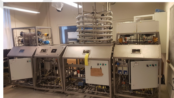
Figure 9: Smart Water Lab at Aalborg University.
