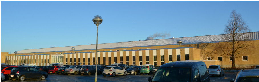
Fig. E.1: Picture from the front side of office building Nord 2.
