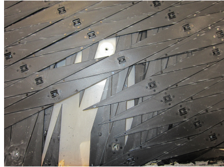
Fig. 1.6: Photo of the internal membrane structure.
