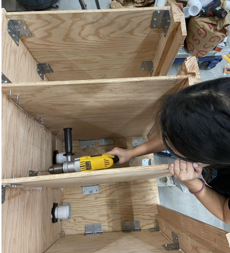
Figure 25. A mid-construction action shot.
