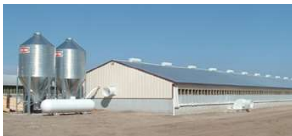
Figure 1.8: Conventional swine production facility ( www.liquidfeeds.com , 2014)
