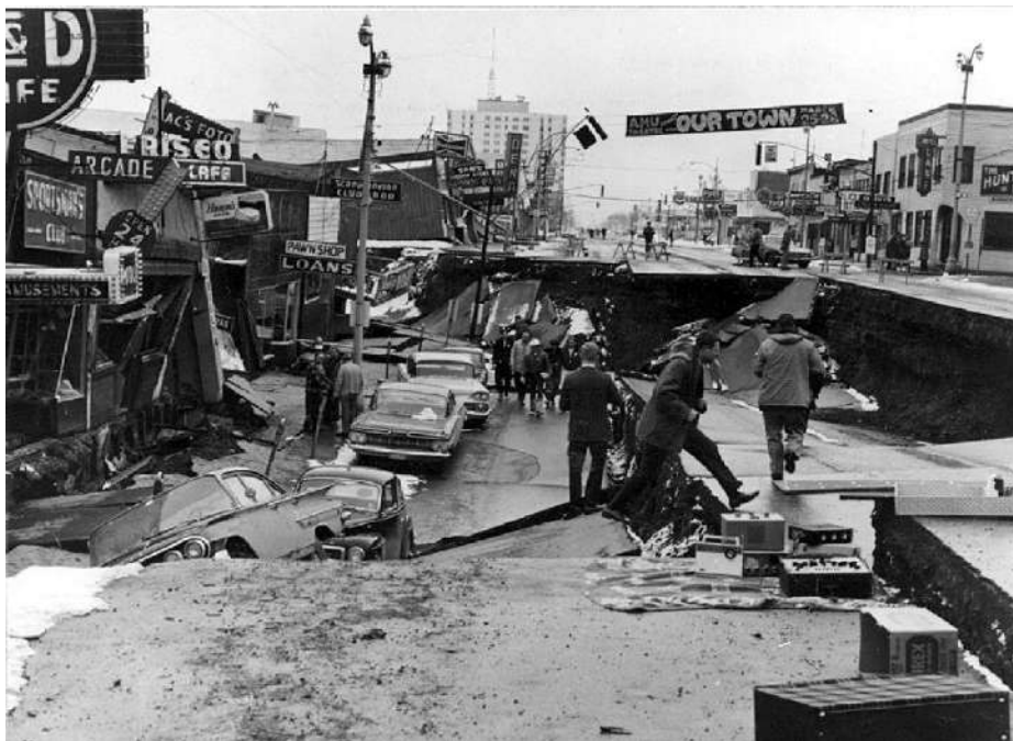
Figure 6.7: The collapse of Fourth Avenue near C Street in Anchorage, Alaska due to a landslide caused by the 1964 Great Alaska Earthquake. Before the tremor, the sidewalk on the left, which is in the graben, was at the street level on the right. The graben came down 11 feet in response to 14 feet of horizontal movement. Photo from the Earth Science Photographs from the U.S. Geological Survey Library (McGregor & Abston, 1995).
