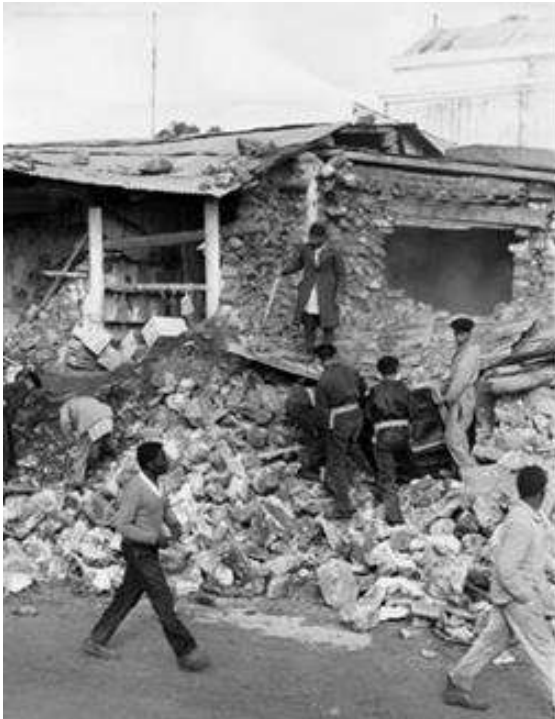
Figure 7.4: An example of damage to a rubble stone and mud house. Photo from Sulfium Forum, 2010.
