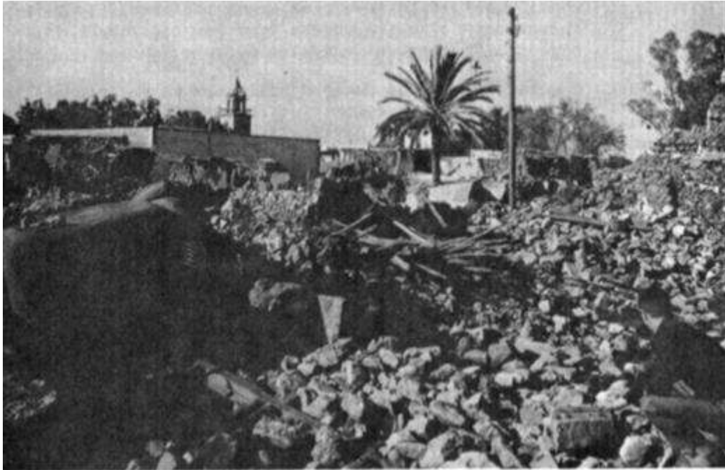
Figure 7.3: The heap of rubble stones in the popular housing area. In the center is the remainder of the fallen roof consisting of wooden rafters. Among the ruins, a building with girders and reinforced concrete columns remain standing though damaged (Minami, 1965).
