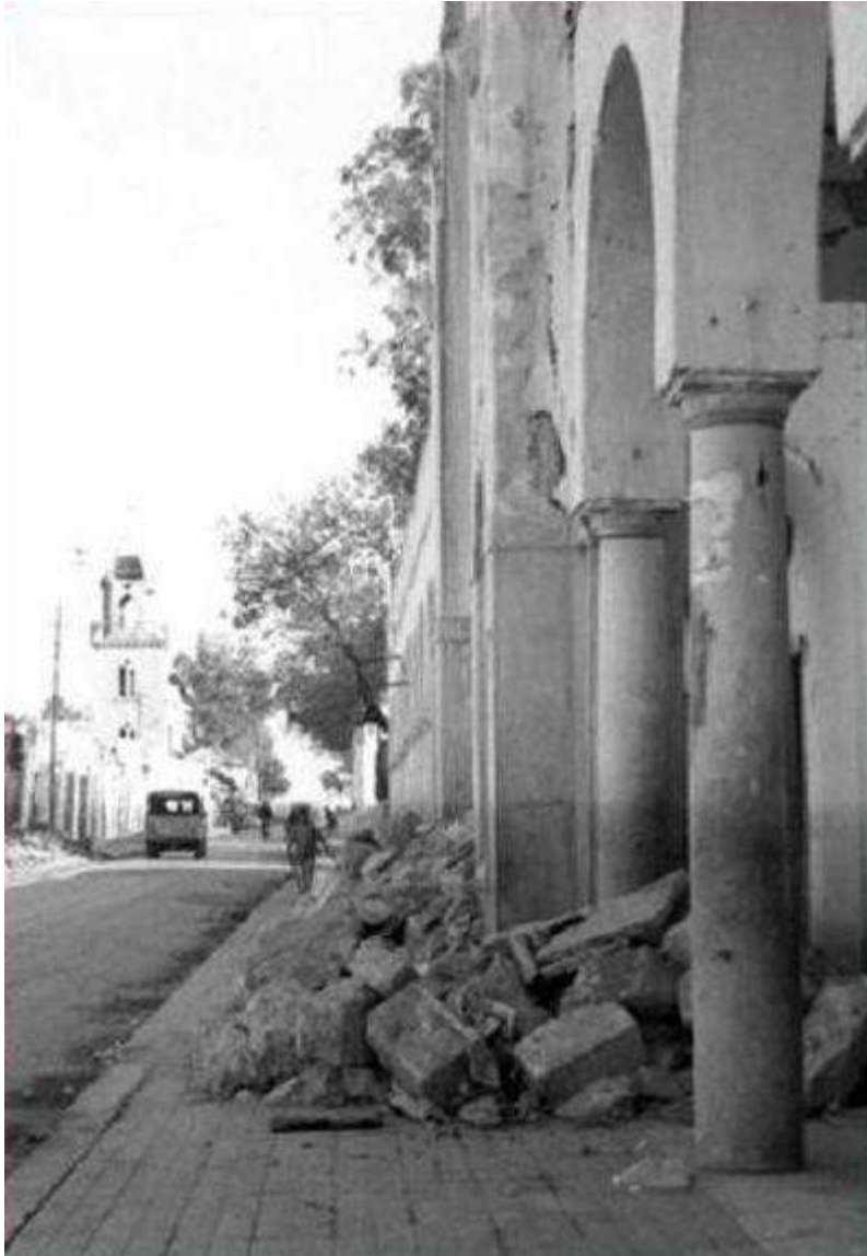
Damage in Al Marj in northeastern Libya from the 1963 earthquake. https://commons.wikimedia.org/wiki/File:El_Marj_earthquake.JPG
