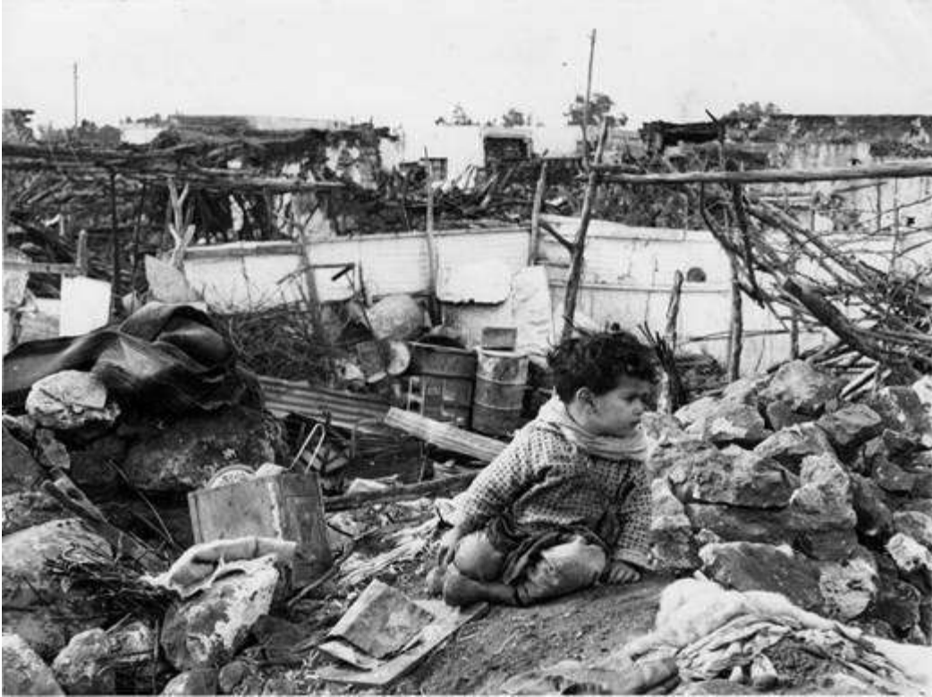
Figure 2.12: The photo shows the damage of the 1963 Al-Marj earthquake (Sulfium Forum, 2010).
