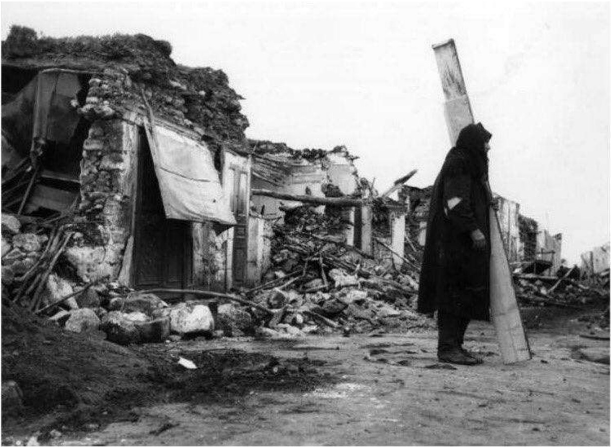
Photograph of the devastation caused by an earthquake in the eastern Libya town of Al-Marj on this day in 1963. https://twitter.com/MaryFitzger/status/966249345812172800
