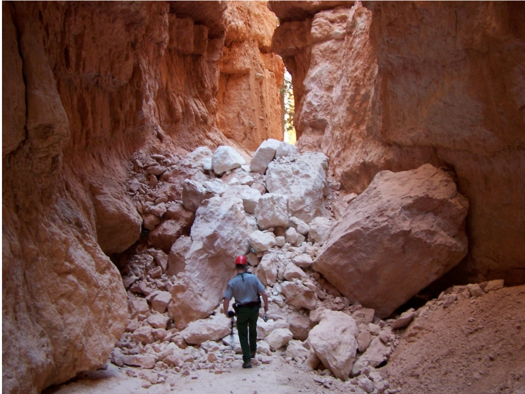
Figure 2.9: 2006 rockfall in the Wall Street section of the Navajo Loop Trail. The rockfall was severe enough that the Navajo Loop Trail remained closed for over a year and the trail had to be rebuilt over debris and, in some cases, completely rerouted (Photo: National Park Service).
