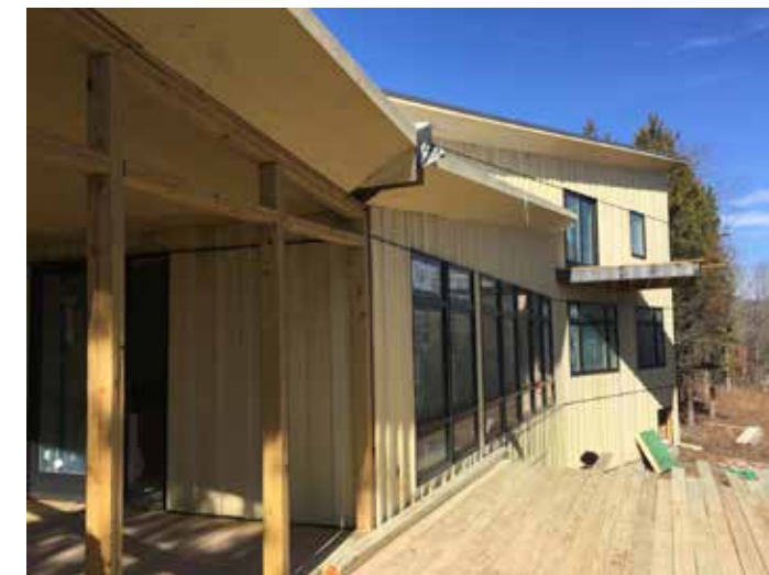
Eagle Point Residence, Garfield (in construction)
