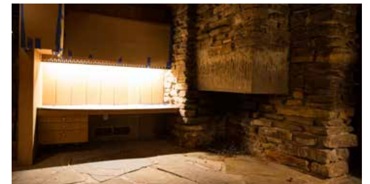
Clockwise from top left: Repairs made to the second floor living area include replacing the ceiling. A view from the front yard during restoration and repair work in fall 2017. A detail of the curved rock wall that runs along the driveway. The house number and another sculpture were part of Jones’ design. One of two built-in desks and the fireplace in the Jones daughters’ childhood bedroom. (All photos by Russell Cothren)
