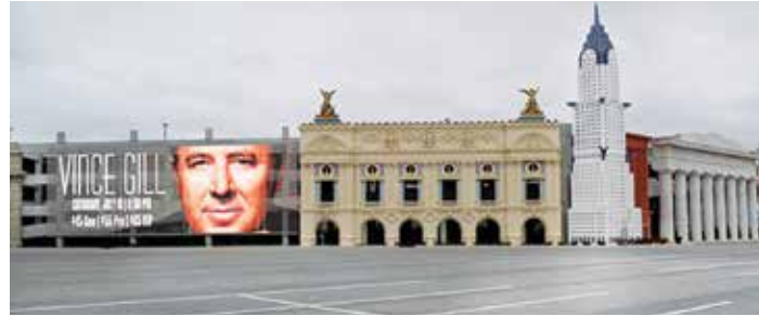
WinStar World Casino Parking Garage. Photo by Gary Dodson
