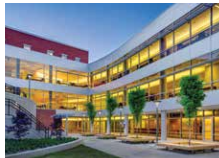
Courtyard at Veterans Administration Medical Center, Fayetteville. Photo by Ken West Photography
