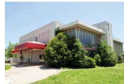
Former bank building, Fort Smith. Photos by Janet Warlick
