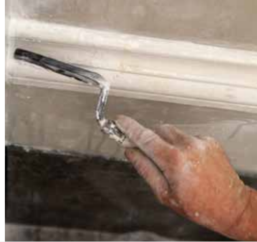
Left: A series of frosted glass fins covers the western facade of the addition. Middle: The arched windows of Vol Walker Hall were restored during the project. Right: A craftsman touches up the molded plaster in the second floor gallery. Opposite page: Left: Glass-walled fire stairs connect Vol Walker Hall and the Anderson Design Center addition. Right: This plan details the landscape strategy for the project.
