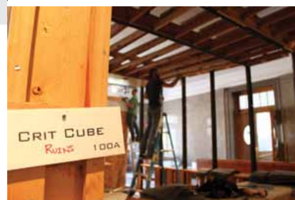
The crit cube's room number was updated during demolition.
