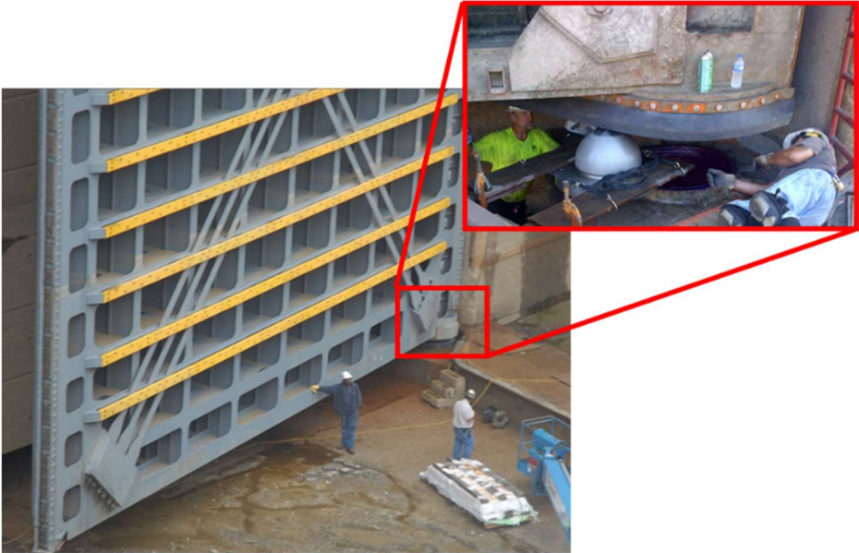
Figure 3. Pintle of a Miter Gate [14]
