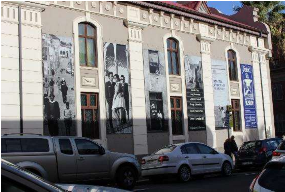
Figure 5.31: Above: Vertical photographic vinyl banners and museum colour blocked signage on the Albertus Street side of the museum building.
