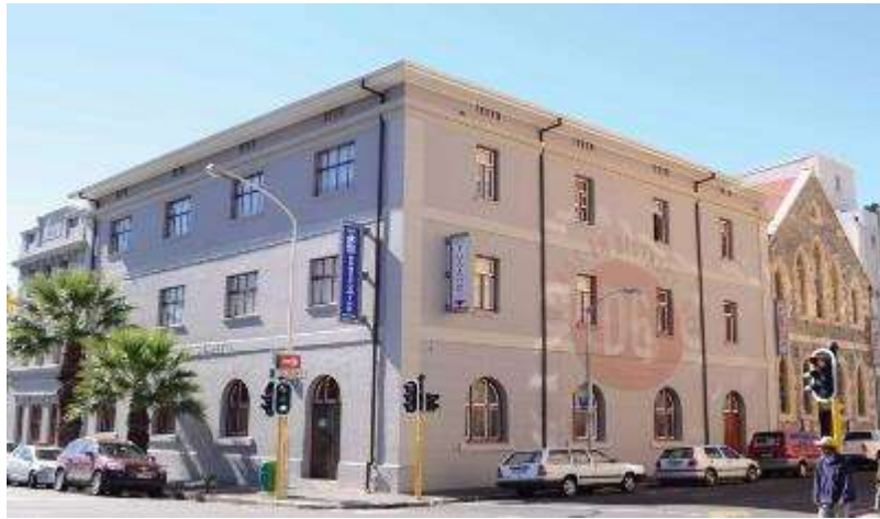
Figure 4.27: The District Six Museum Homecoming Centre in Buitenkant Street, once the Saks Futeran wholesale business occupying 5 interconnected buildings. The warehouse building on the left and the Fugard Theatre building on the right link to the main double-story warehouse building. Photograph: HH-R
