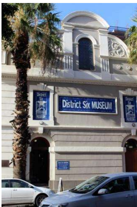
Figure 5.30: Color-blocked blue and white signage engineered to sit within the historic plaster detail of the Buitenkant Street Museum façade created more visual unity and legibility. Photograph HH-R.
