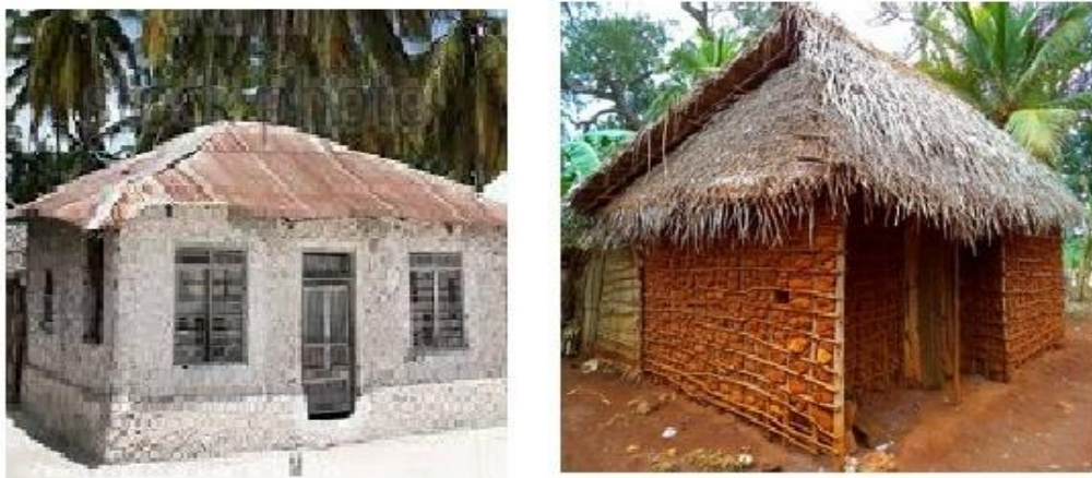
Figure 1.2: Traditional houses built with beach sand (left) and soil (right).
