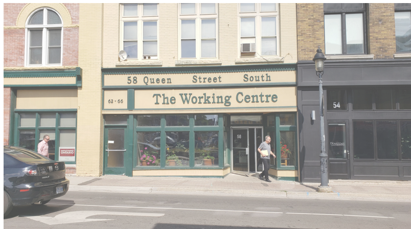
Fig. 19. The Working Centre, 58 Queen Street South, Kitchener, ON.
