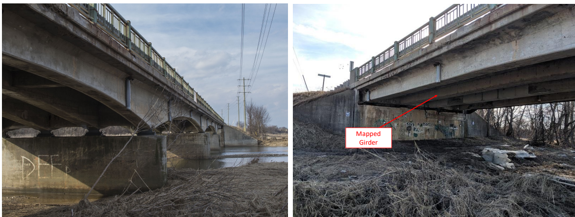
Figure 5.1: Northfield Drive bridge over the Conestogo River. (Photos by: Nicholas Charon)
