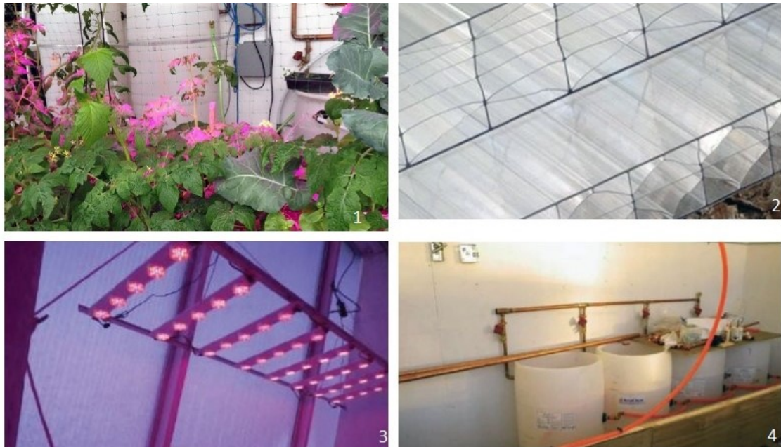
Figure 26. Greenhouse at Yukon, Canada (1. Inside of the greenhouse, 2. Glazing material, 3. LED for lighting, 4. Heating and Power Station) (Walden Labs, 2015)
