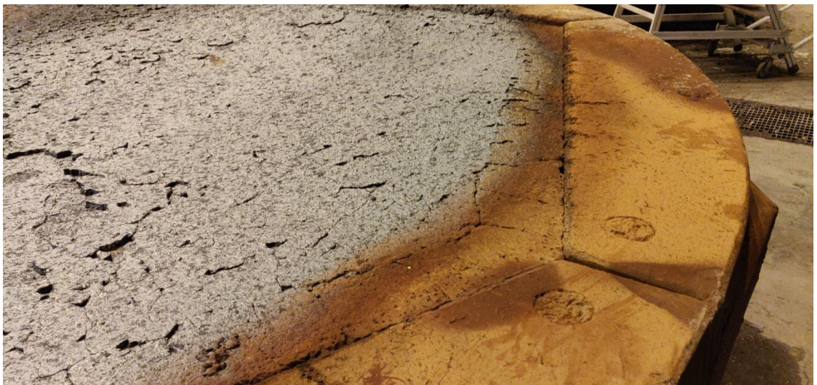
Figure 41. Minor cracks can be seen circling near the edge of the monolithic lining after 200 heats.
