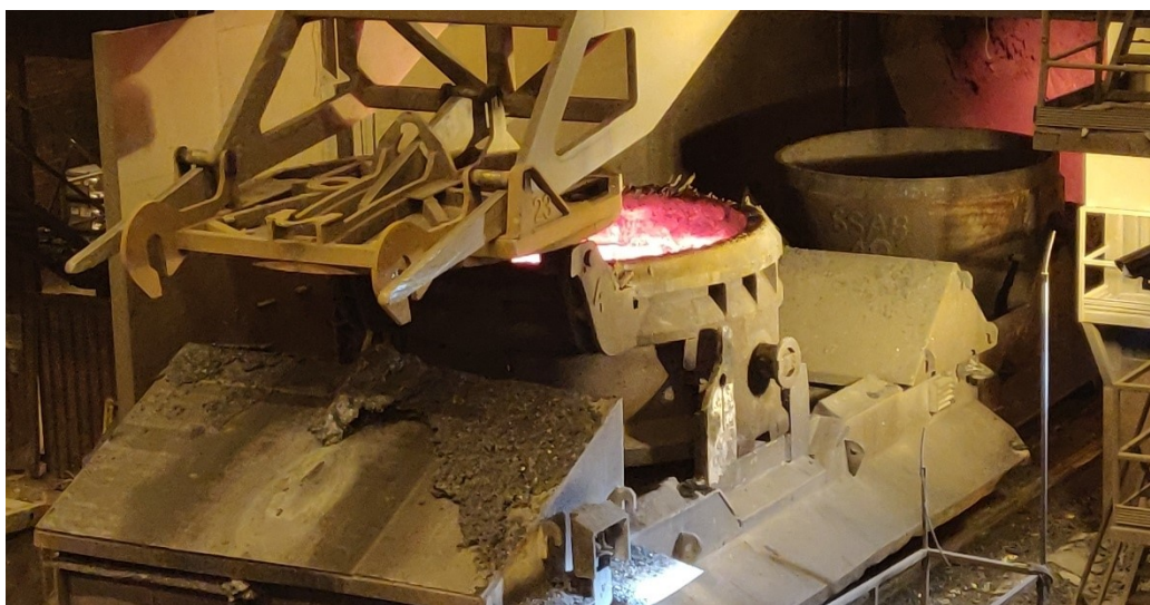
Figure 13. Lid stored on the rack near the converter (BOF).
