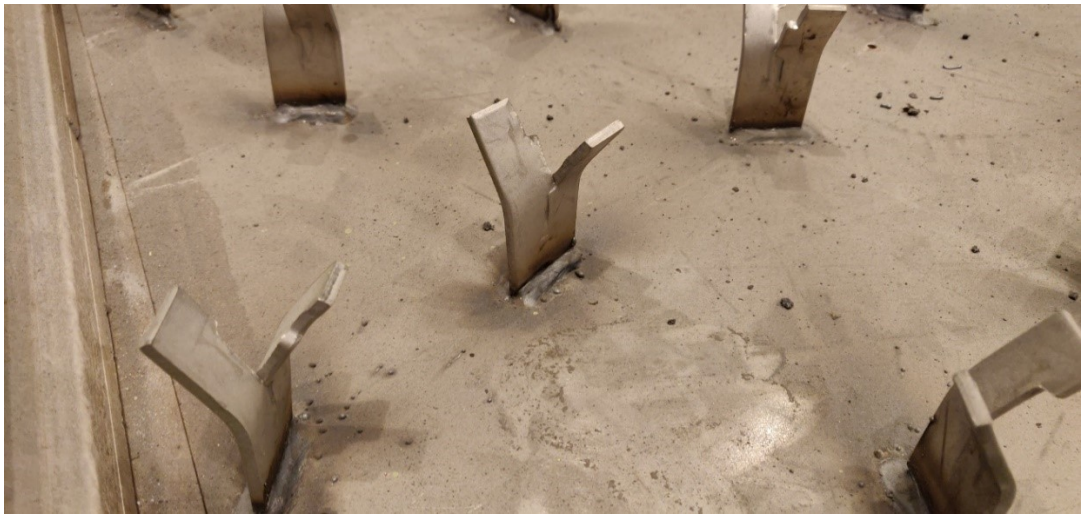
Figure 10. Metal anchors welded on the back plate of the lid.
