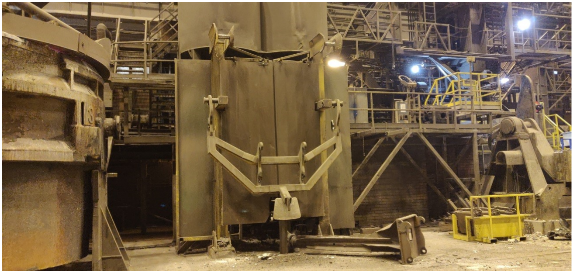
Figure 15. Devices at desculling station. Lid grabbing tool for a loader is hanging from the lid holder and deskulling anchor is on the ground.
