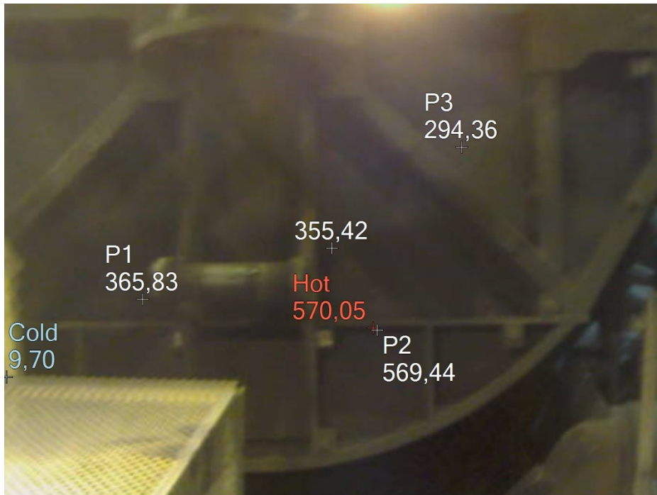
Figure 49. No visible defects observed on the backplate.
