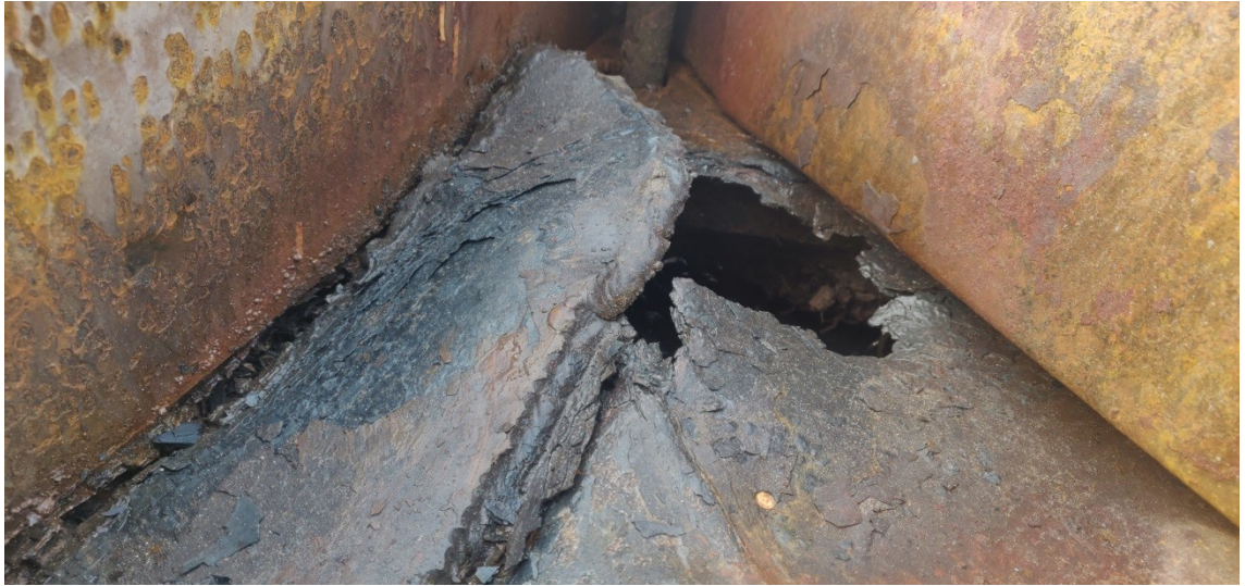
Figure 35. Continuous exposure to heat causes plate to lose its shape and rupture.
