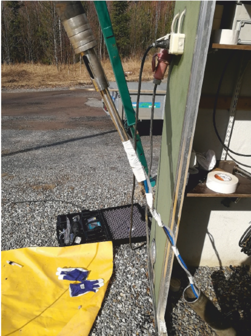
Figure 14. Installation of the packers in the drillhole during the field work. The figure shows the lower part of the upper packer, pressure probe (blue probe), flow-through probe (white) and stainless-steel rod.
