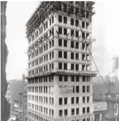
Reinforced concrete structure
