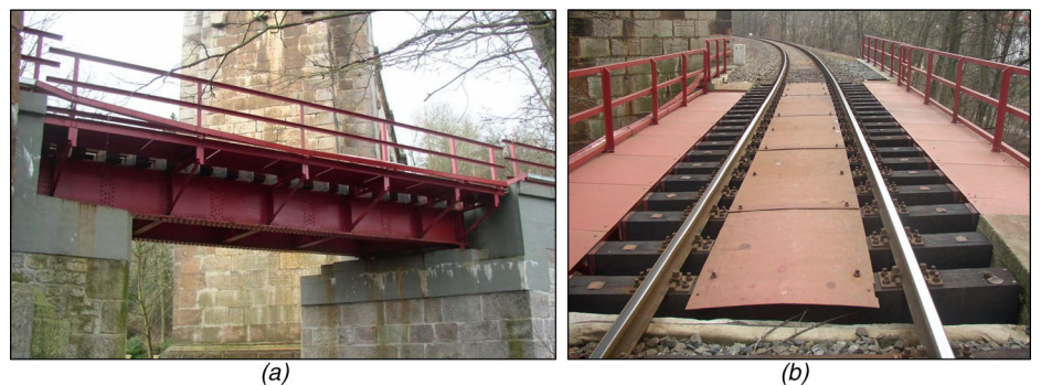
Fig. 2: Railway bridge: (a) longitudinal view; (b) view of the superstructure
