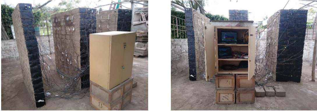
Figure 4: Place of installation and continuous monitoring center of three adobe walls.
