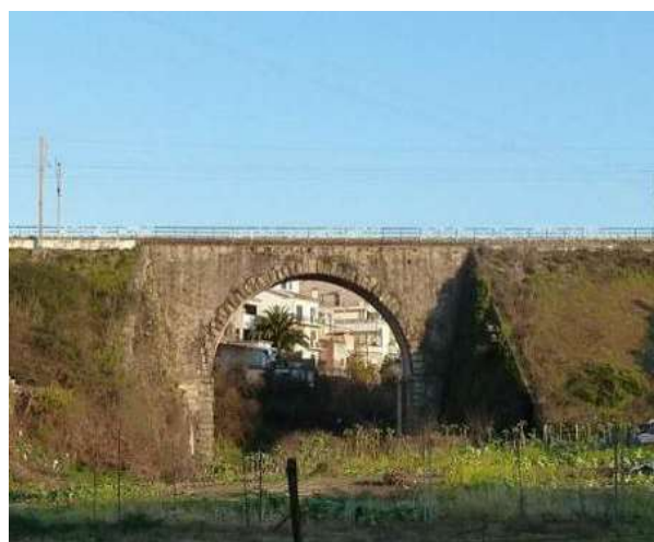
Figure 1. Leça railway bridge
