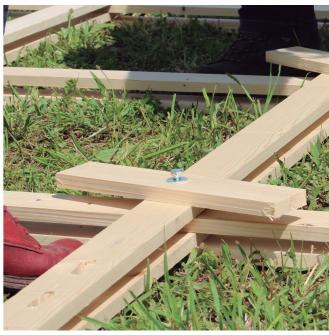
Figure 12 a, b. Gridshell Construction
