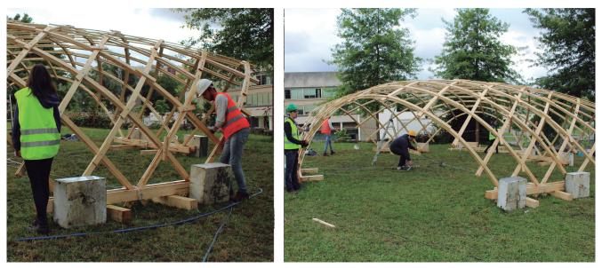
Figure 17 a, b. Gridshell Construction
