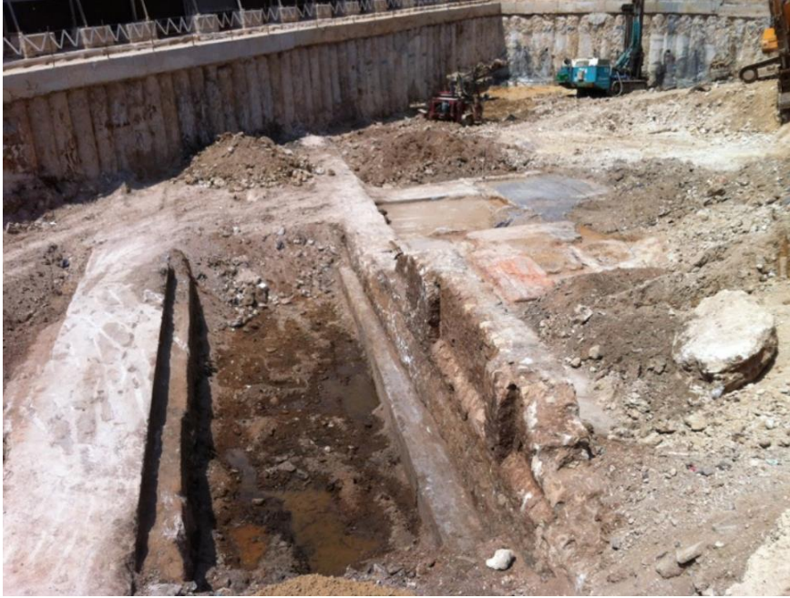
Figure 86: Old structures found during the excavation phase
