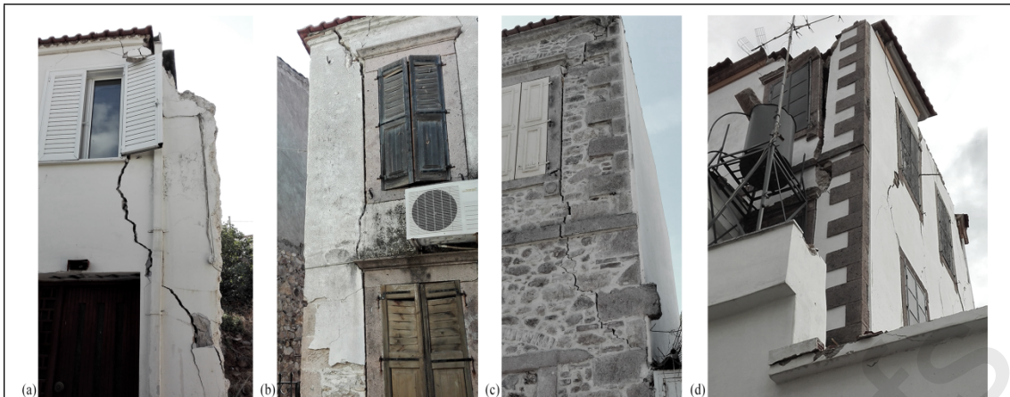
Figure 14. (a)-(d) Weak connection of transversal walls, due to the presence of openings at the corner proximity.
