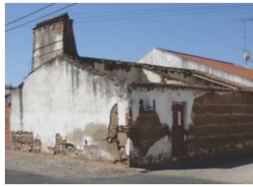
876 Fig. 1. Rammed earth constructions in Portugal: (a) Alentejo region (in red); (b) examples of typical dwellings 877 (Silva et al. 2018b)
