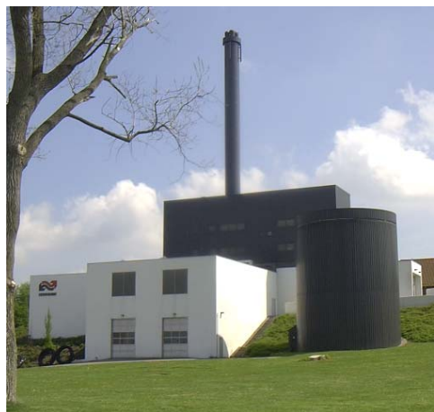
Fig. 11. Hot water storage tank in a DH station
