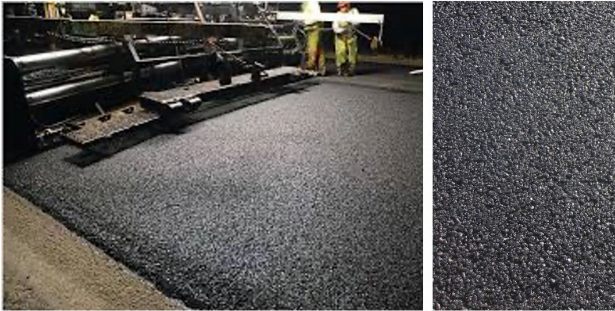
a) Behind Screed of Spray Paver
