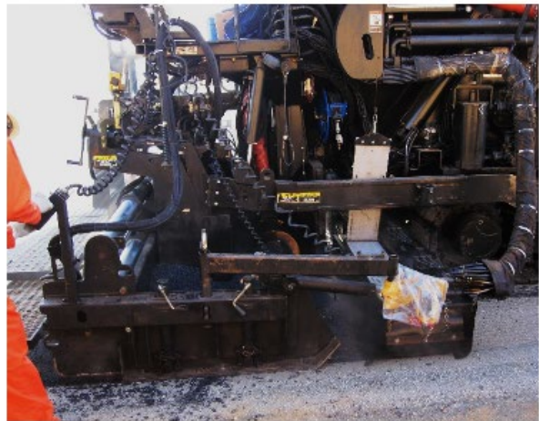
b) Spray Paver Screed
