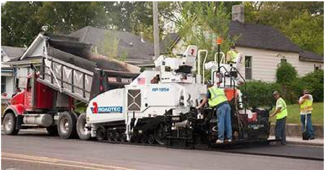
Figure 12. Roadtec Paver Paving Residential Street with Thin Asphalt Overlay Surfacing
