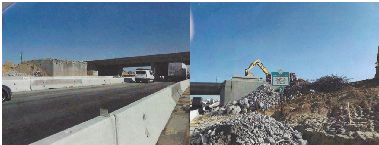
Figure 2. RCA from Demolition of a 50-Year-Old Bridge
