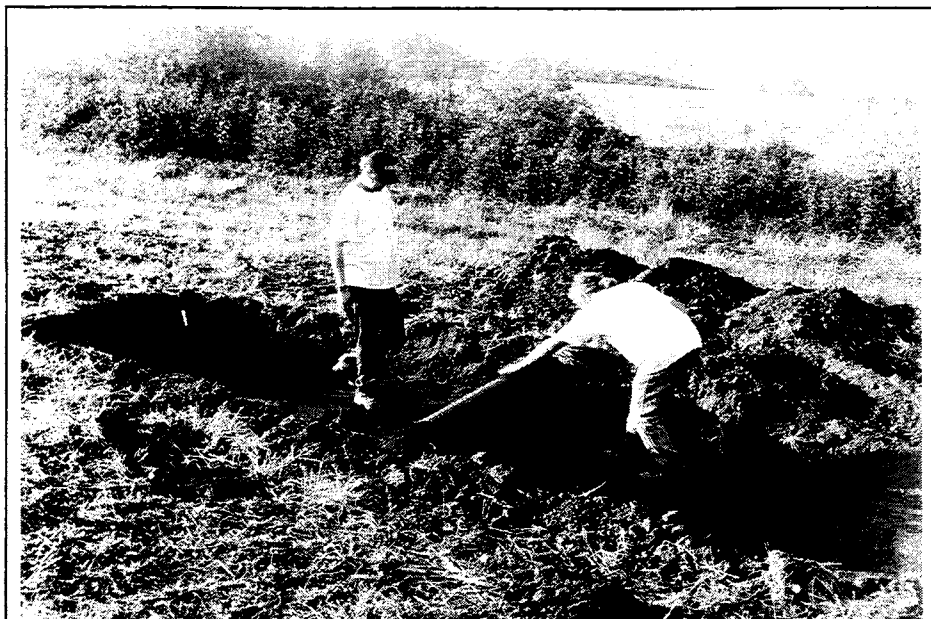
Figure 13. Installing filter fabric after cleaning and plotting a trench.
