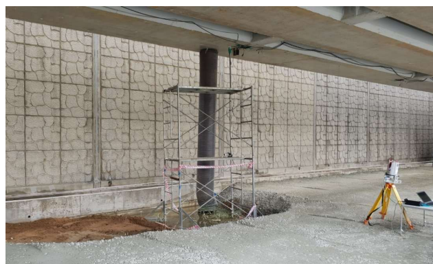
Figure 55. Preparation for the underpass pavement.
