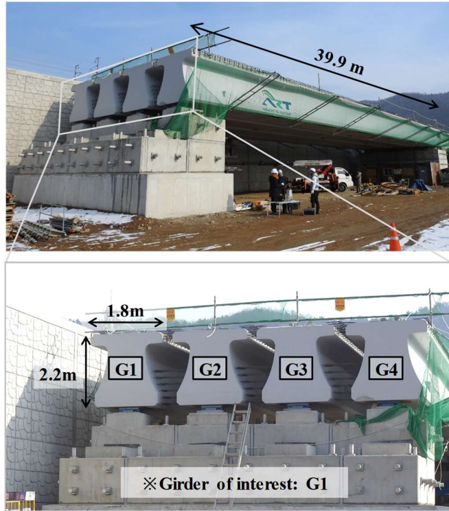
(a) Bridge under construction (December 19, 2017)
