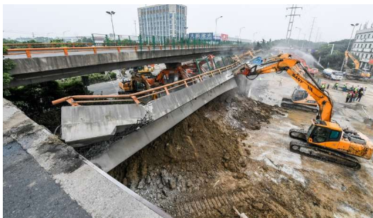
(c) The National highway 312 in China, a concrete bridge built in 2005
