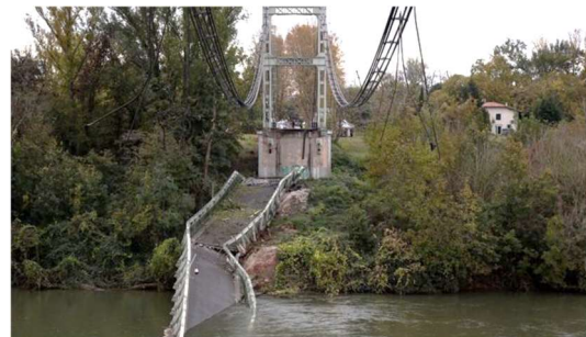
(d) The Mirepoix bridge in France, a suspension bridge built in 1931
