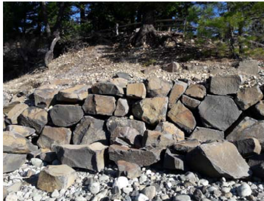
Figure 40: Rip-Rap near Speelyi Beach, Cle Elum Lake. Photograph by Michael Horner.
