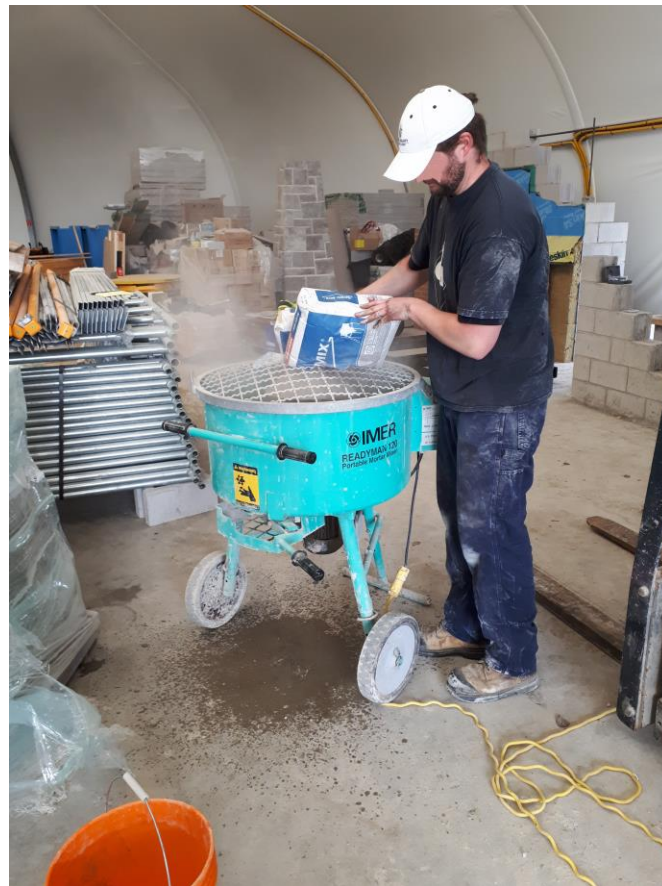
Figure 2.3: Mechanical mixing of Type S Spec Mix mortar.
