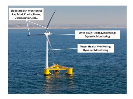
Figure 2.11: Sensors for WTHM.
