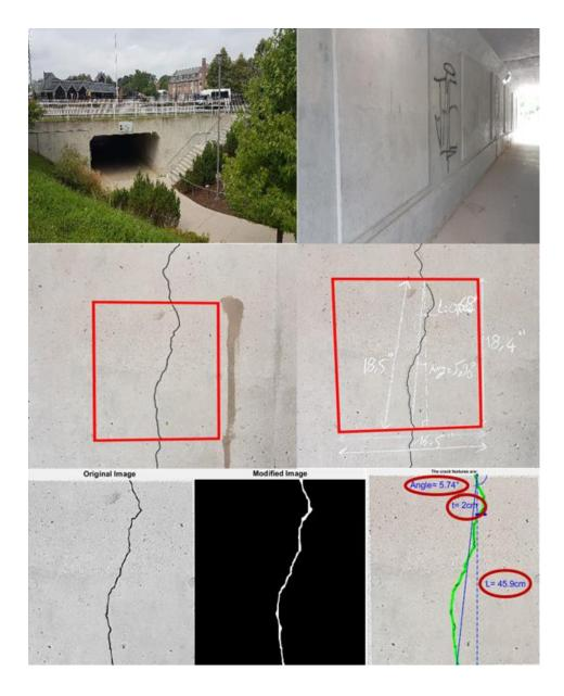
Figure 3.21: Calculation of Crack Features of a Damaged Reinforced Concrete wall.
