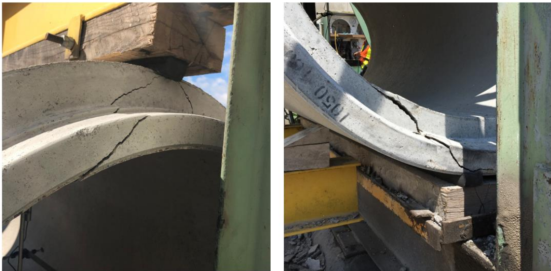
Figure 3.9-Diagonal Tension Cracks at Applied Load (Left) and Support (Right).
