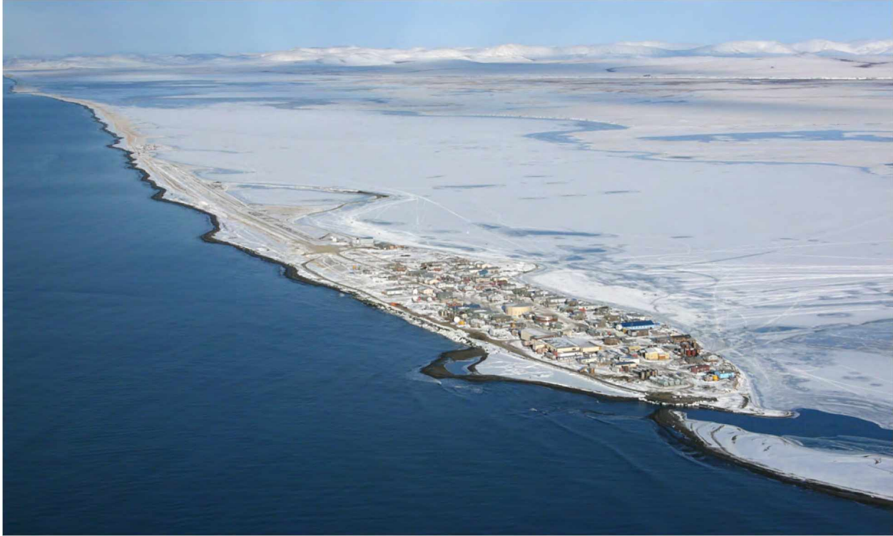
Figure 3-3 The remote northwest Alaska community of Kivalina. Kivalina is at risk from erosion and rising sea levels. During the study period, the Division of Subsistence conducted three comprehensive subsistence survey projects in Kivalina: 1983, 1992, and 2007. In smaller communities like Kivalina (2010 population, 374), research designs usually called for a census rather than a probability sample.
