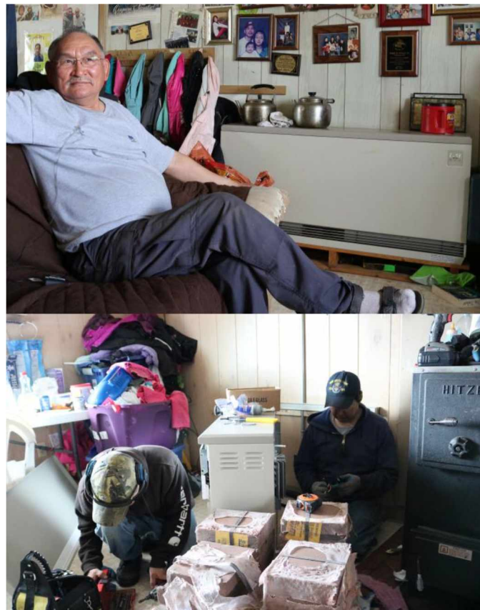
Figure 3.7. Community member sits in front of the electric thermal stove installed in his home (top) and local workers prepare ceramic bricks for installation in a electric thermal stove in another residence (bottom) in Kongiganak, Alaska. Electric thermal stoves are used to store excess wind energy as heat in ceramic bricks which displaces a portion of oil heating in individual residences. Source: Alaska Center for Energy and Power, University of Alaska Fairbanks.
