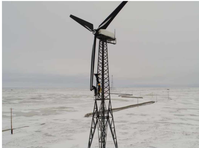
Figure 3.10. Locally trained technicians reset a tip brake on a 95 kW wind turbine after a strong wind caused the brakes to deploy in Kongiganak, Alaska. Source: Alaska Center for Energy and Power, University of Alaska Fairbanks.
