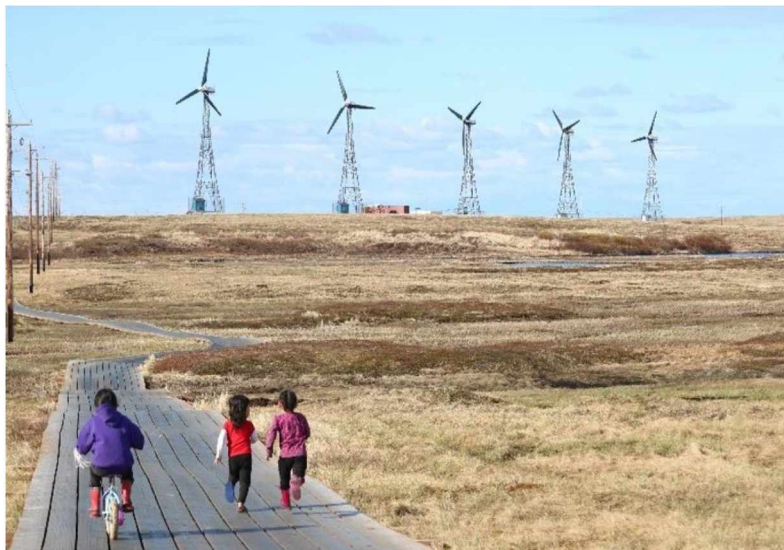
Figure 3.8. Five 95 kW wind turbines are installed in Kongiganak, Alaska which help to displace a large proportion of more costly diesel electric generation and oil heating in residences through the use of electric thermal stoves. Source: Alaska Center for Energy and Power, University of Alaska Fairbanks.
