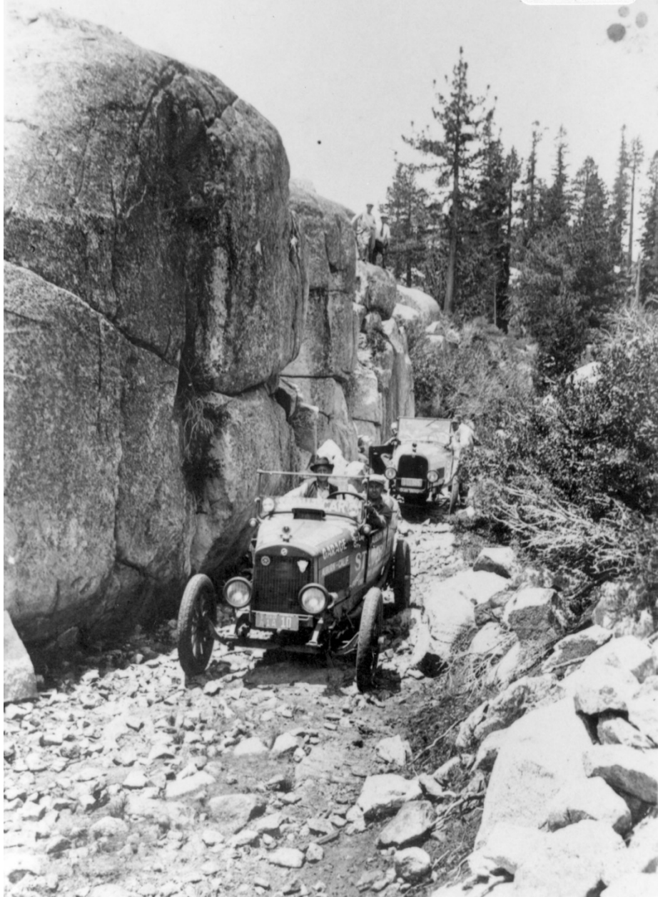
Figure 3.2. The two custom Studebakers that make the first motorized trip across the entirety of the Rubicon Trail in June, 1926. In this photograph, the two cars are passing through the “Sluice Box,” through which motorists descend into Rubicon Springs from the West. Photo Courtesy of the El Dorado County Museum.
