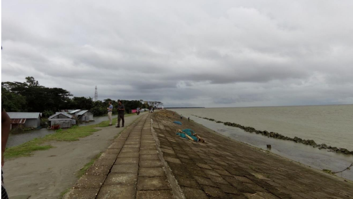
Figure 2.4 Revetment in Ramgati (Source: Author)
