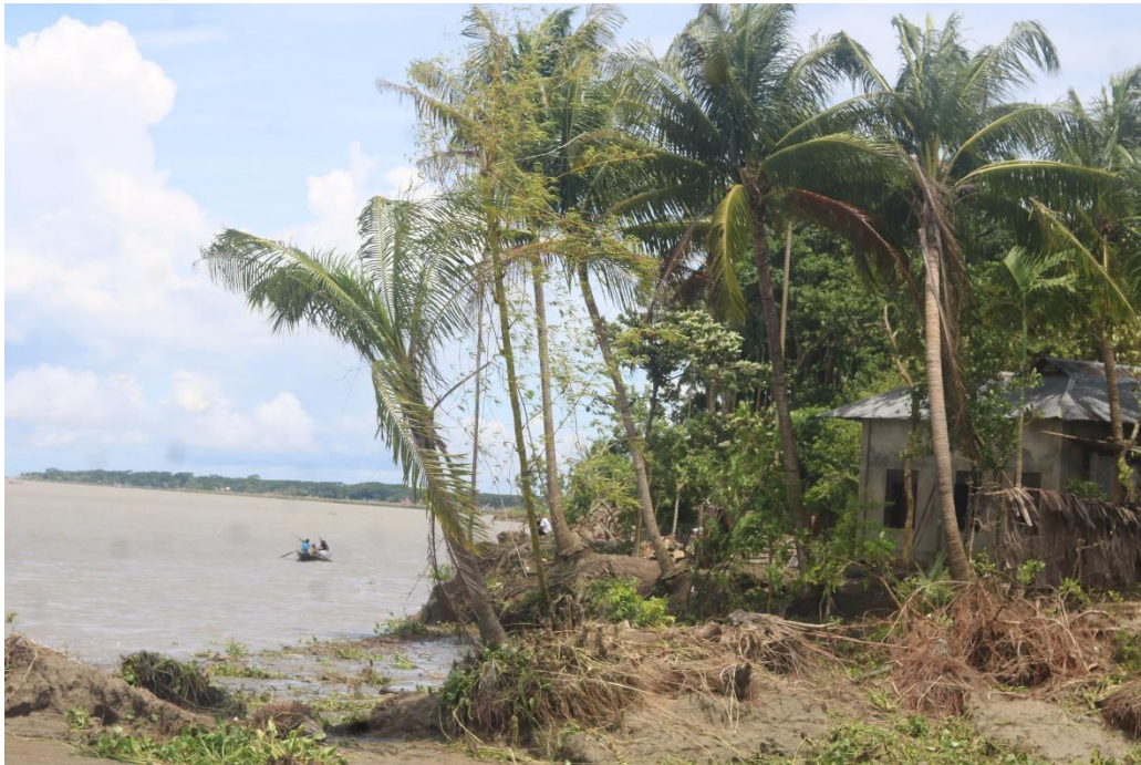
Figure 5.4 Riverbank Erosion In Ramgati (Source: Author)
