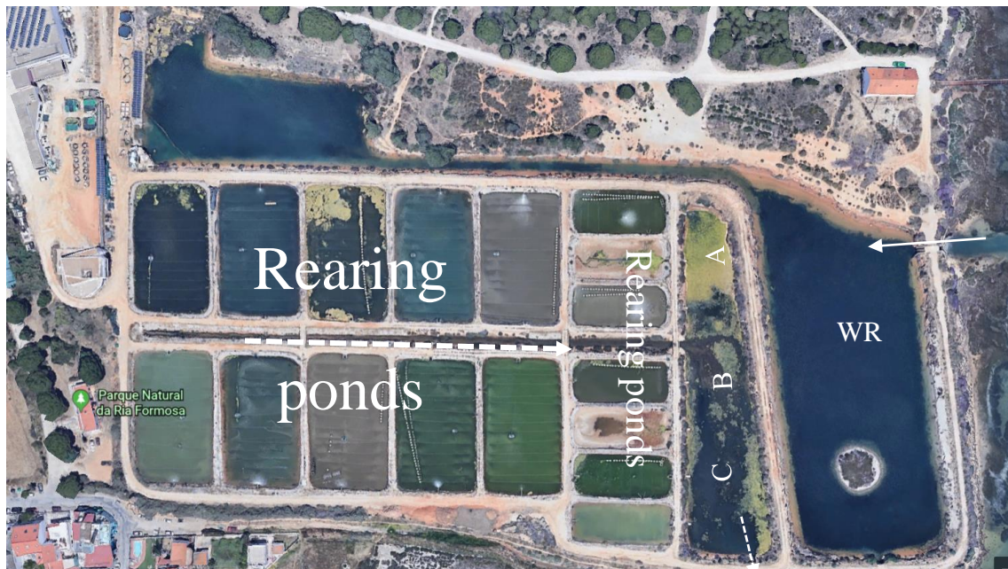
Figure 2. The research station production area, composed of water reservoir (WR) with connection to the Ria Formosa, 17 rearing ponds and lastly, where samples were performed, settling pond divided in three areas (A to the right of the rearing tanks outflowing water channel; B area proximal to the channel; C area to the left of the channel). Solid arrow represents inflowing water and dotted arrows outflowing water. Source: Google earth V 9.3.94.1.
