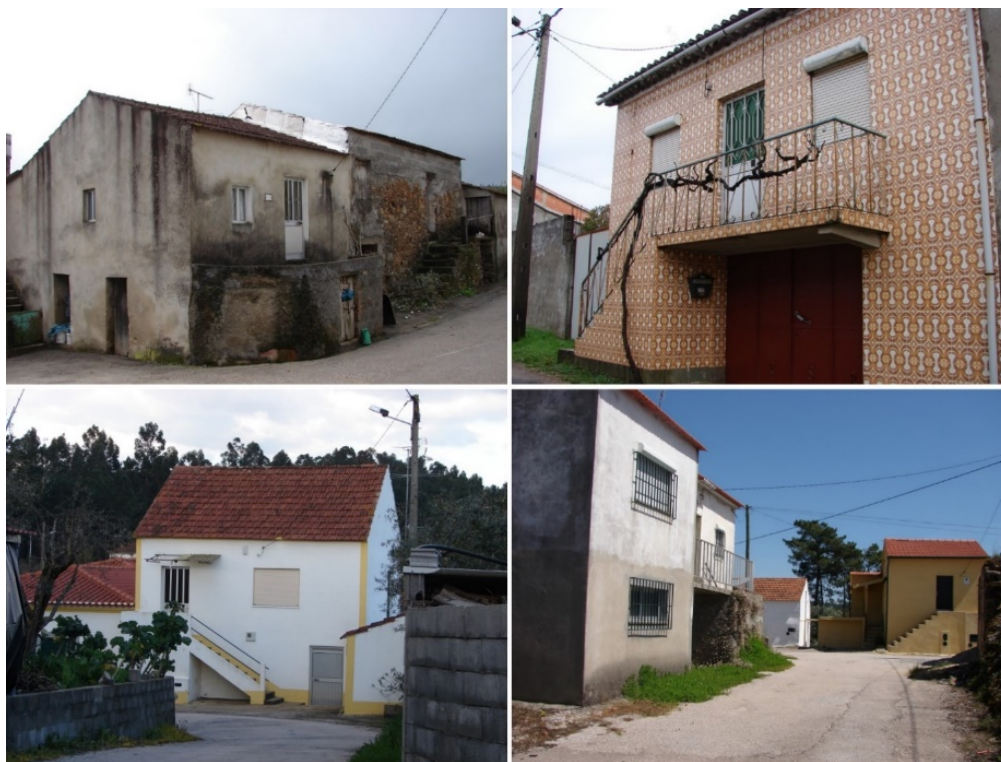
Figure 6. Traditional houses with two floors and exterior staircase, already with changes, Cernache do Bonjardim. Above: left – Sambado; right – Alcobia. Below: left – Casal da Madalena; right – Escudeiros
