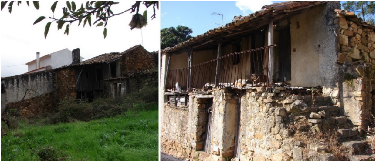
Figure 4. Traditional houses with two floors and with porch external staircase, Cernache do Bonjardim. Left: Sambado; right: Porto dos Fusos
