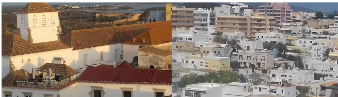
Figure 2. Traditional flat rooftops in the city of Faro.
