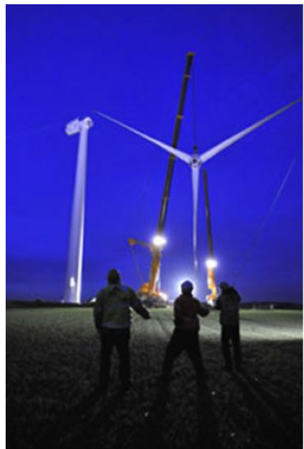
Turbines Siemens Bonus 1.3MW, Hub Height 49m, Rotor diameter 60m; Blade length: 31m
