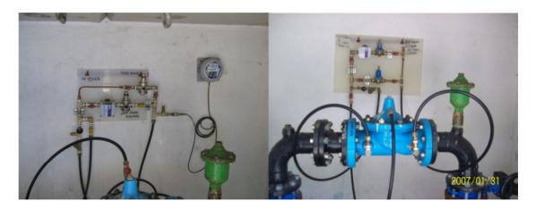
Figure 3.7: Dual pilot time control system connected to PRV
