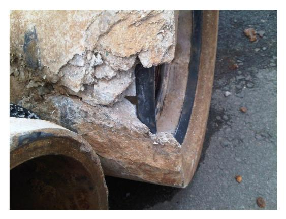
Figure D.10 AC collar failure due to faulty rubber seal
