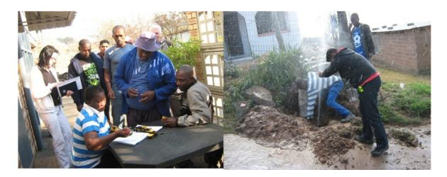
Figure 3.26: Category B Plumbing Leak Detection and Repair. (Photo courtesy of Mr Chris Otto, 2010)
