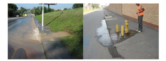
Figure 3.13: Examples of Typical Leaks within eThekwini Municipality
