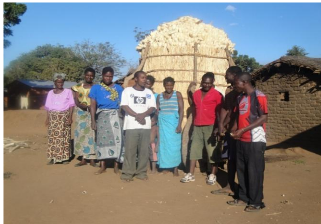
Figure 2.1: Maize storage structure in Chinguluwe Extension Planning Area (EPA), Salima district
